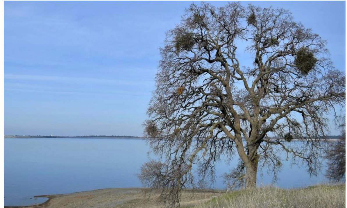
The lake side of the Mormon Island Auxiliary Dam looking west
