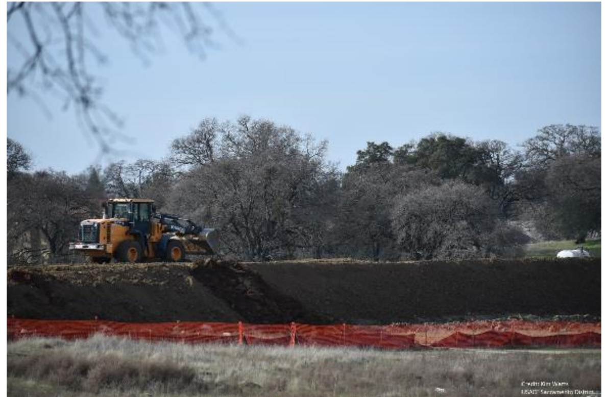
Dike 8 construction looking south
