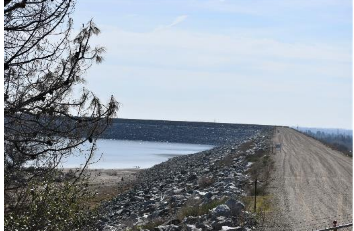
North end of the Right Wing Dam, looking south.
